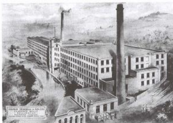
Above: Print used on certificates by the Fine Cotton Spinners & Doublers Association of Clarence Mill in 1920, showing the two former swing bridges.
